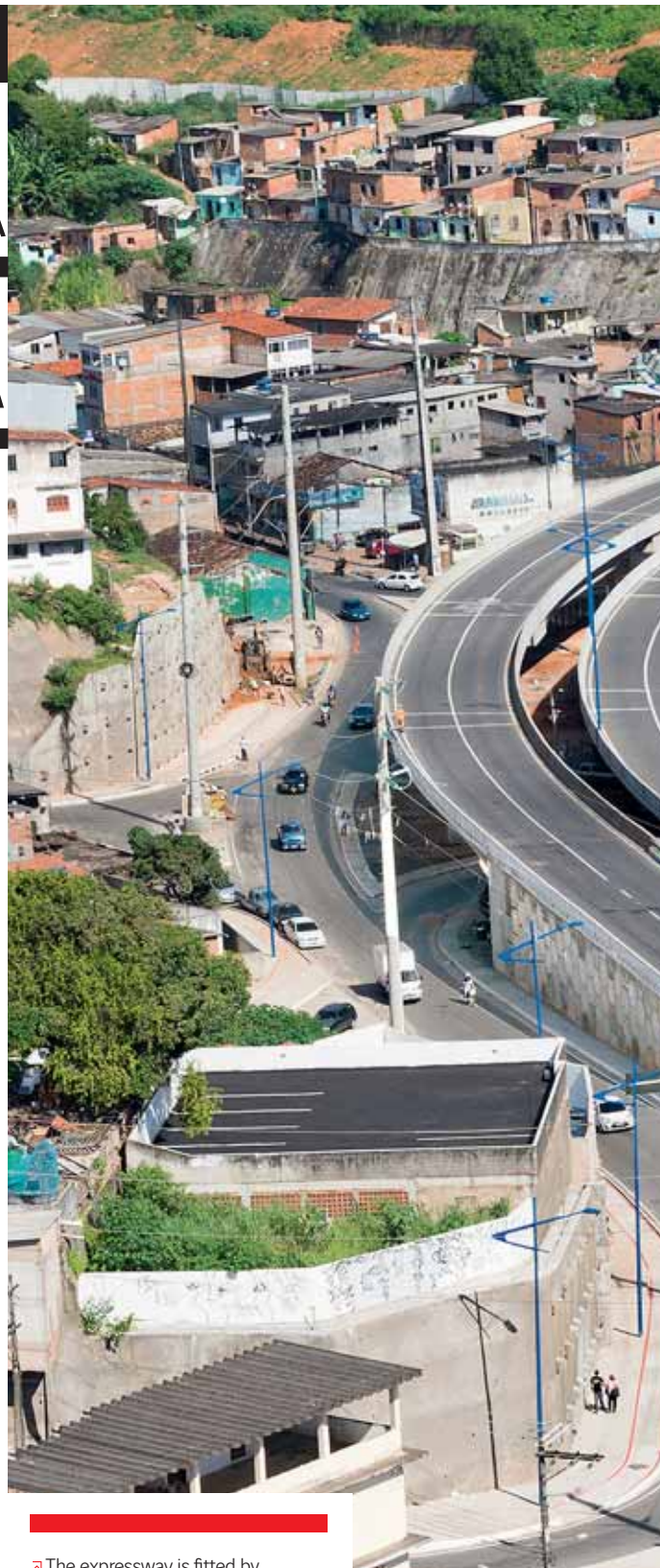
➤ The expressway is fitted by twenty structures in TerraClass® walls, totaling 19,030 m 2 .
