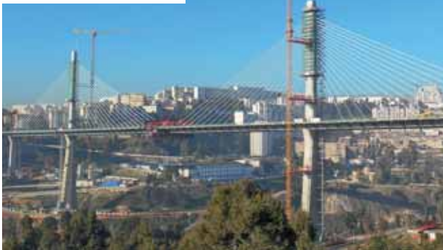
THE CONSTANTINE VIADUCT, THE SECOND AFRICAN CABLE-STAYED BRIDGE
