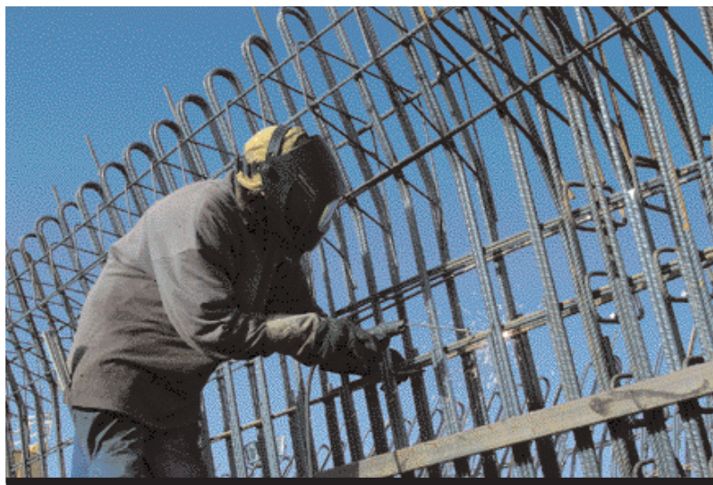
Manufactured using B50 self-placing concrete to simplify casting into the mould, the U beams are composed of 10.5 t of passive steel, 64 m³ of concrete and 5.4 t of prestressing steel.
