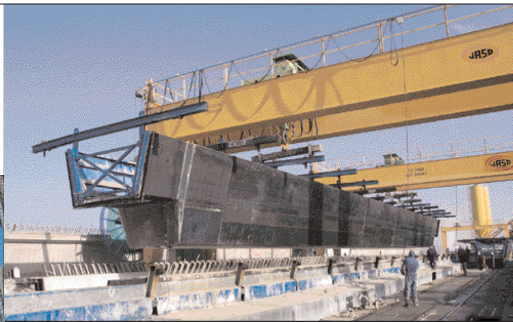
Manufactured using B50 self-placing concrete to simplify casting into the mould, the U beams are composed of 10.5 t of passive steel, 64 m³ of concrete and 5.4 t of prestressing steel.
