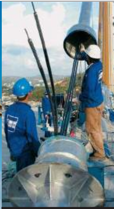
A central layer of stay cables, narrower protective pipes in special colours: three solutions to help the structure blend into the panorama.
