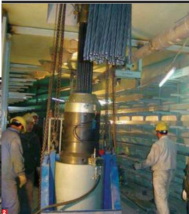
1. Construction of the foundations of the containment vault for the new EPR European reactor in Olkiluoto. 2. Anchor point for the vertical prestressing for a containment vault in China.
