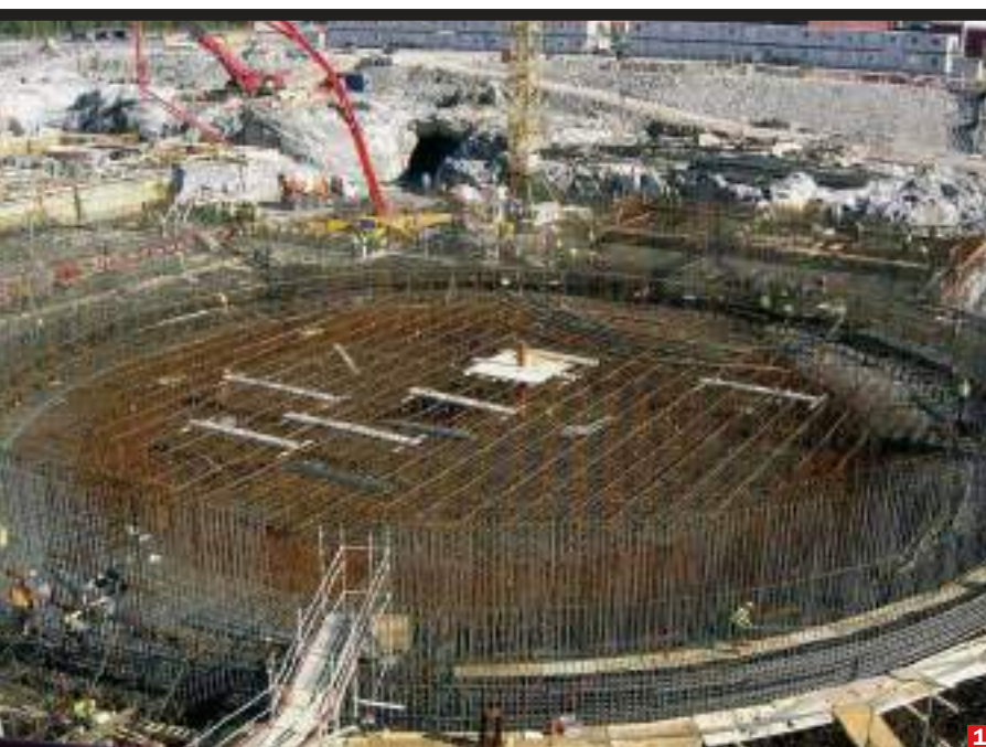
1. Construction of the foundations of the containment vault for the new EPR European reactor in Olkiluoto. 2. Anchor point for the vertical prestressing for a containment vault in China.
