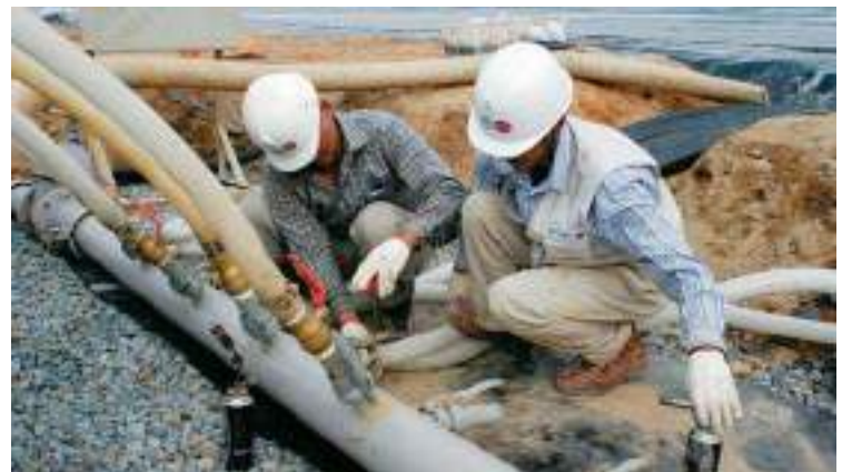
The underground network of 1,300 km of drains connected to pumps will allow for the soil to be restructured within 12 months.
